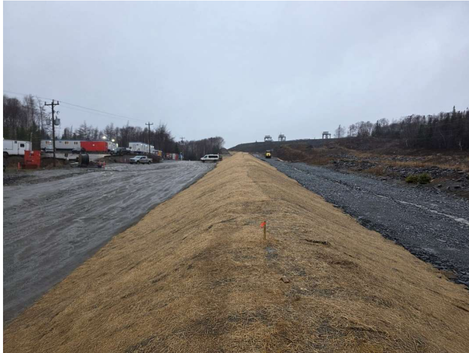
Figure 1: Completed Penstock – Replacement Section
